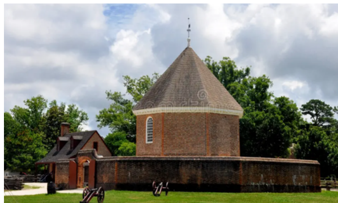
Williamsburg Power Magazine
