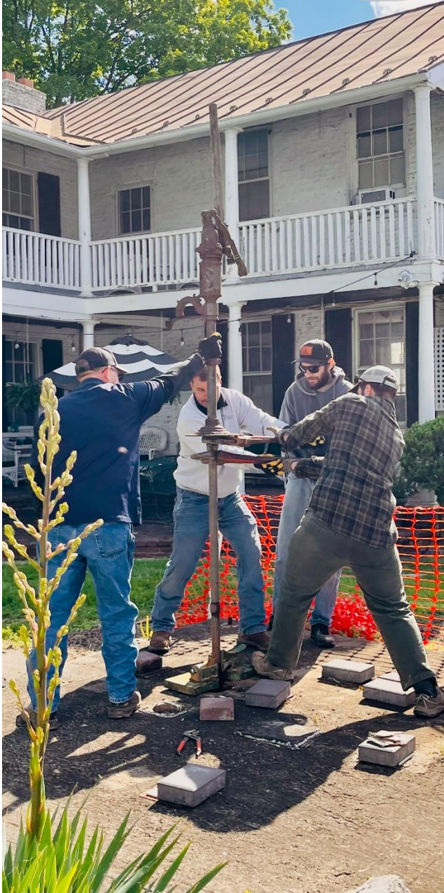
Well Hand Pump Removal by Runyon Pump & Well Service May 2025
