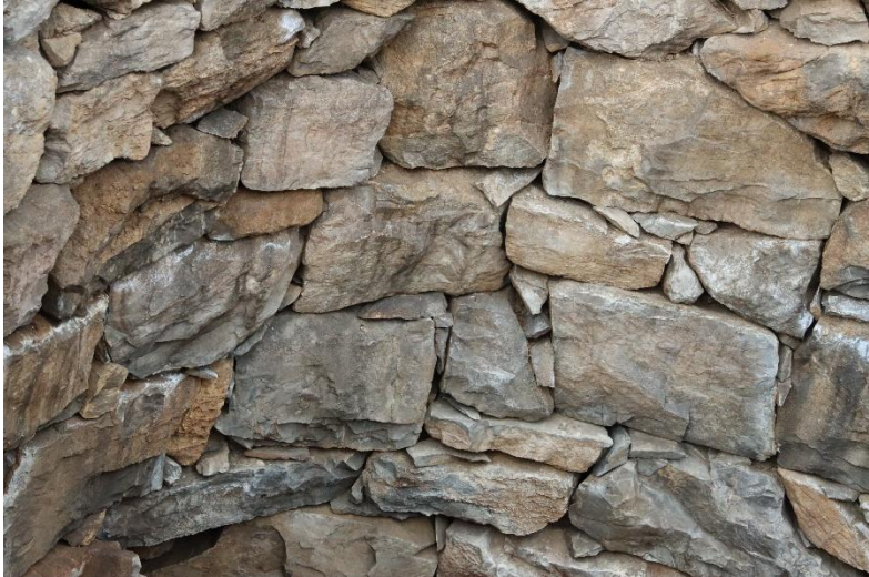
Dry Laid Stonework with Chinking Stones
