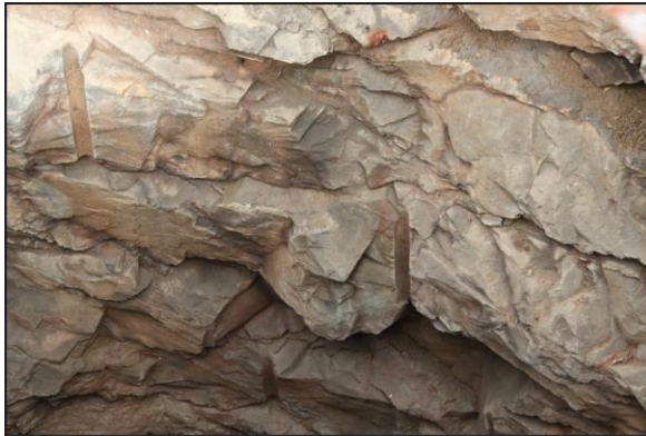
Auger and Blast Holes
