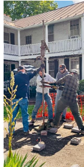
Runyon Pump & Well Service removing the well's hand pump
