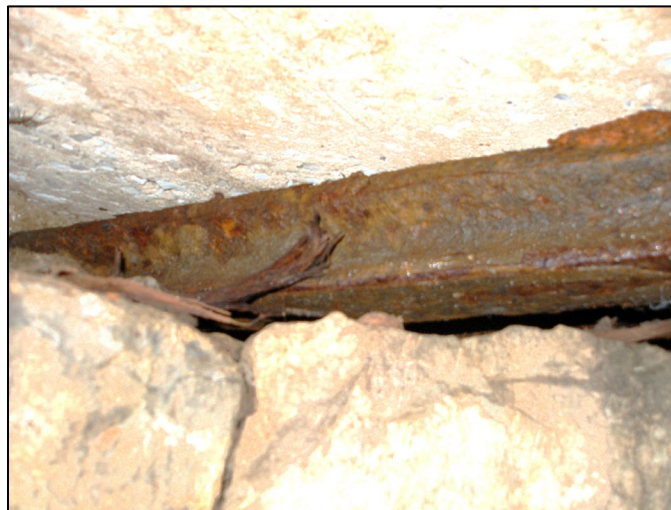
Figure 12: Photographic image. Another view of some of the five (5) layers and the short section of railroad track. Photograph provided by The French & Indian War Foundation, October 2023.
